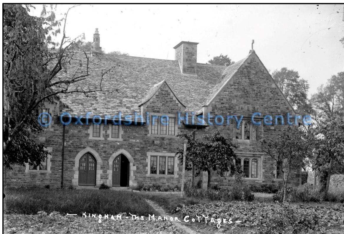
Manor Cottages, built in 1922 on the site of New College's earlier manor house (OHC, POX0193916). Note the reused medieval cylindrical chimney.
