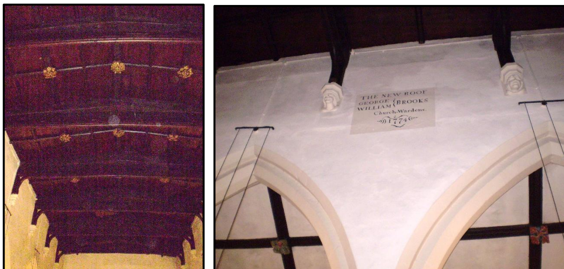
The nave roof (left) repaired in 1774 by that year's churchwardens (right). Reuse of old timbers made it 'look not so well as before', prompting the rector to ceil it at his own cost. Note the glimpse of the north aisle roof (right) repaired in 1769.
