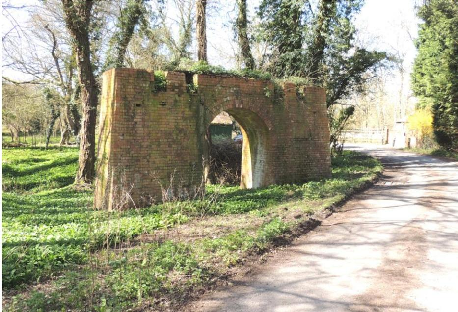
*Figure 1 One of two arches that supported the ramp that transported clay to the pug mill. The arches are the only substantial remains of the Slades Bridge brickworks still standing in 2013.*
