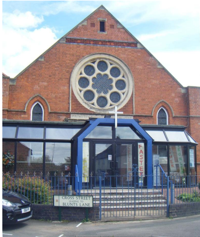
Figure 3: Moat Street Methodist Chapel (formerly Primitive Methodist)
