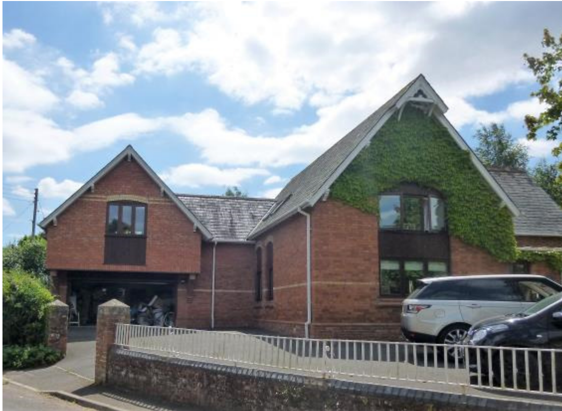
Former school Bradford on Tone
