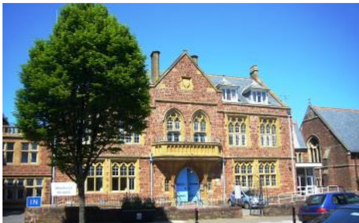
Minehead hospital shortly before closure
