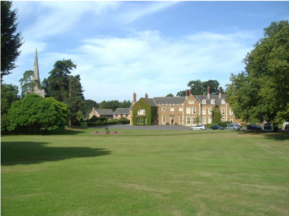
Brooksby Hall, south elevation
