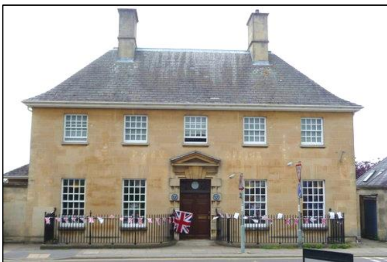
The former post office at No. 13 West Street.
