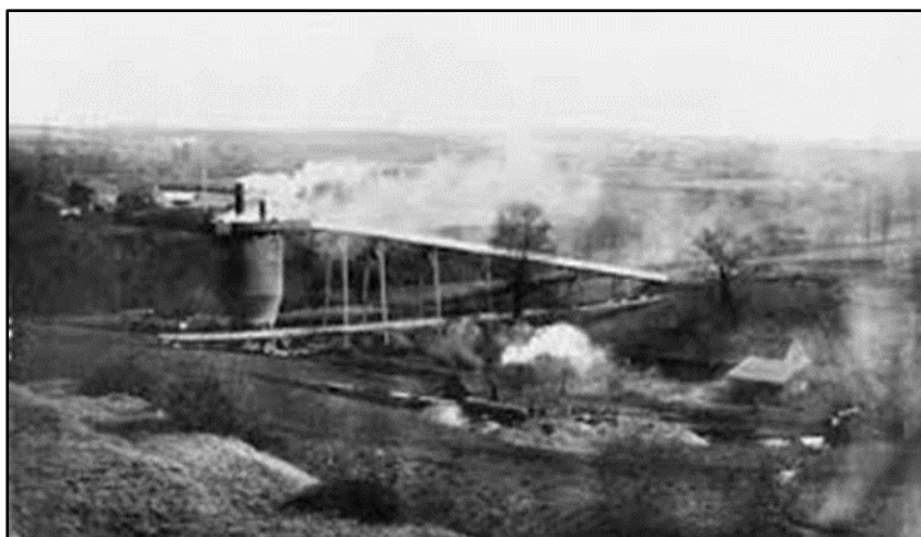
Hook Norton ironstone works: one of the calcining kilns in operation.
