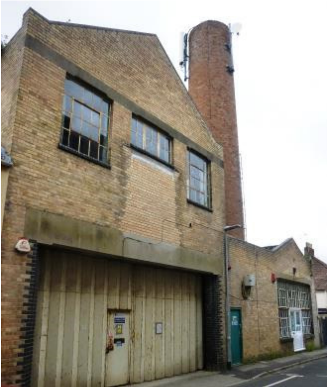
Factory chimney used as a communication mast at Princes St, Taunton. The scar marks the site of a bridge to the main Viney Street factory.
