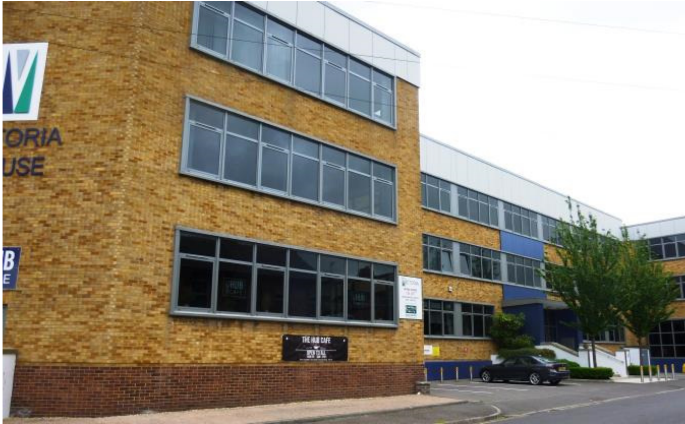
Former Van Heusen collar and shirt factory, Taunton Victoria Street frontage.
