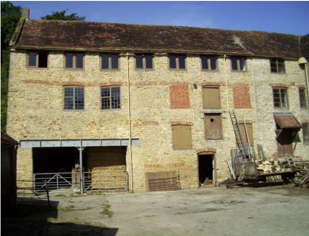
Gant's Mill, Bruton, addition of c. 1812
