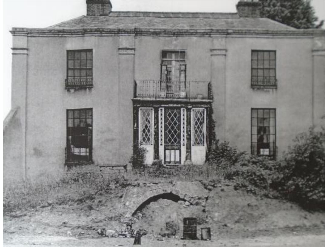
The garden front c. 1970 showing signs of considerable subsidence and a buttress appears to have been built against the left-hand corner. Also visible is the vault under the former conservatory. The roof has been altered and the attic window removed but the balcony survives. The garden has been destroyed. SWHT
