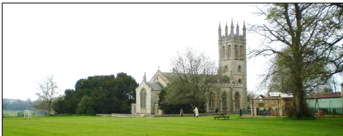
Churchill parish church (built 1825–6) from the north-east.
