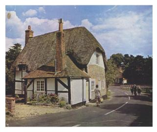
date. The 2-storey house has two rooms with axial spine beams and an end stack and there are many re-used timbers. Both buildings have the small-panel framing and short, straight braces typical of the early 17<sup>th</sup> century and, although they were built
