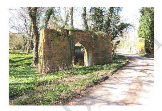
Figure 1 One of two arches that supported the ramp that transported clay to the pug mill. The arches are the only substantial remains of the Slades Bridge brickworks still standing in 2013.
